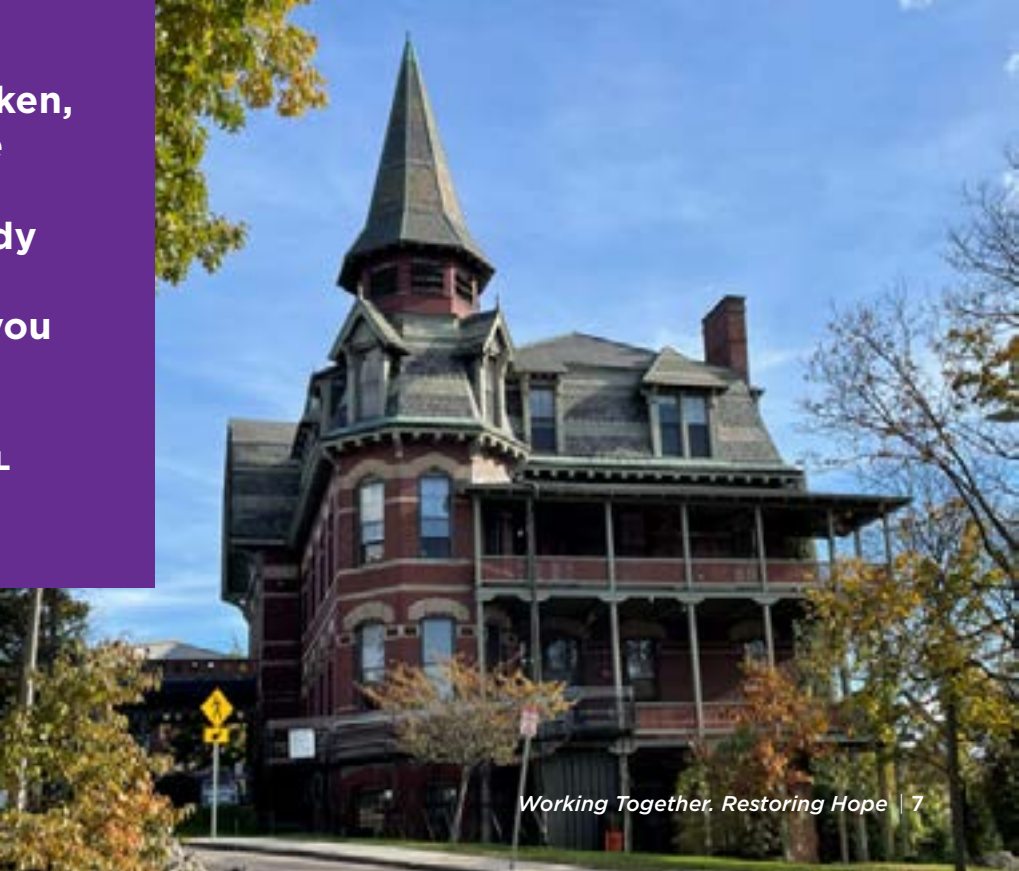
The historic "Z" Building, named after Dimock pioneer Dr. Marie Elizabeth Zakrzewska, will be renovated to create Boston's first post-detox CSS program for men.
